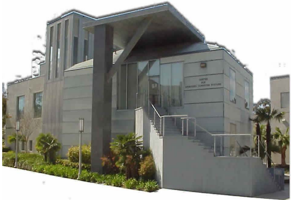
CECS Research Facility
