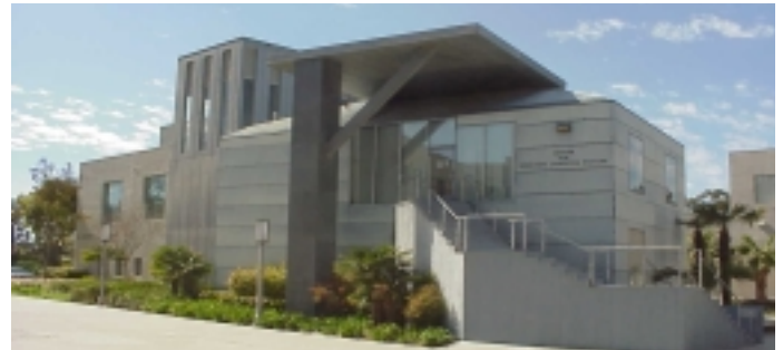
CECS Research Facility
